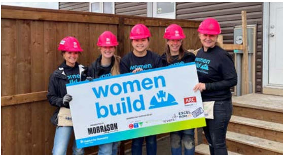
ARC employees helping to build homes at the Women Build 2023 event for Habitat for Humanity
